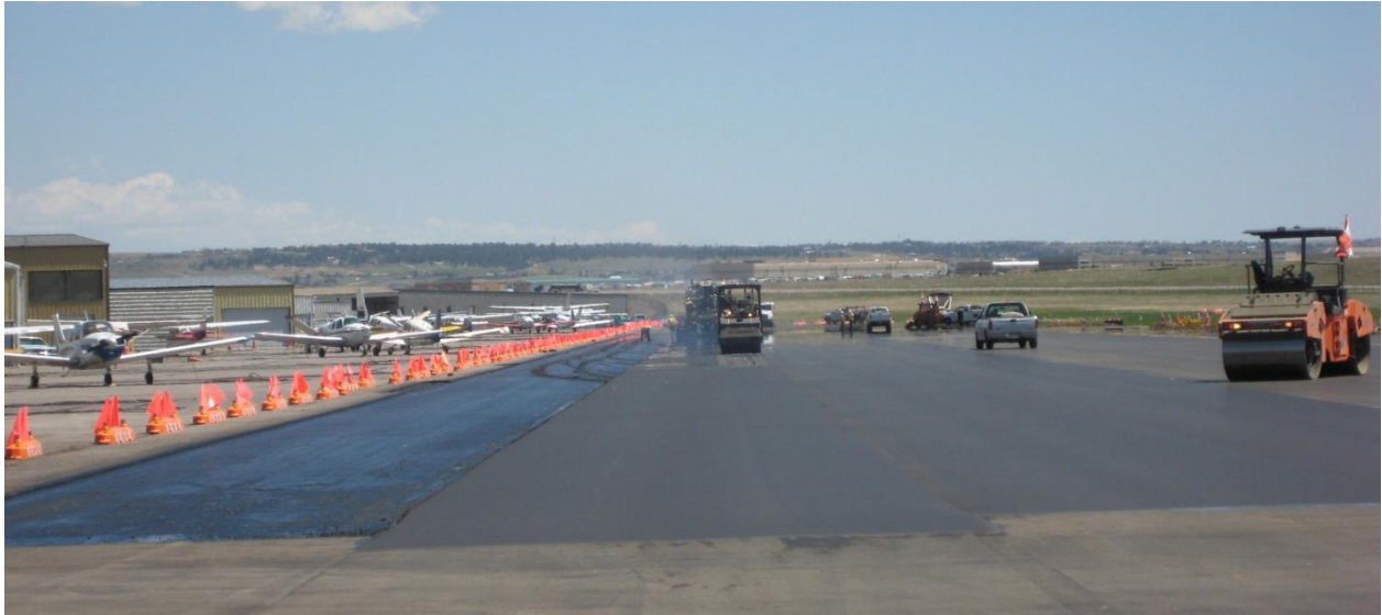
Figure 2-9. Low Profile Barricades
