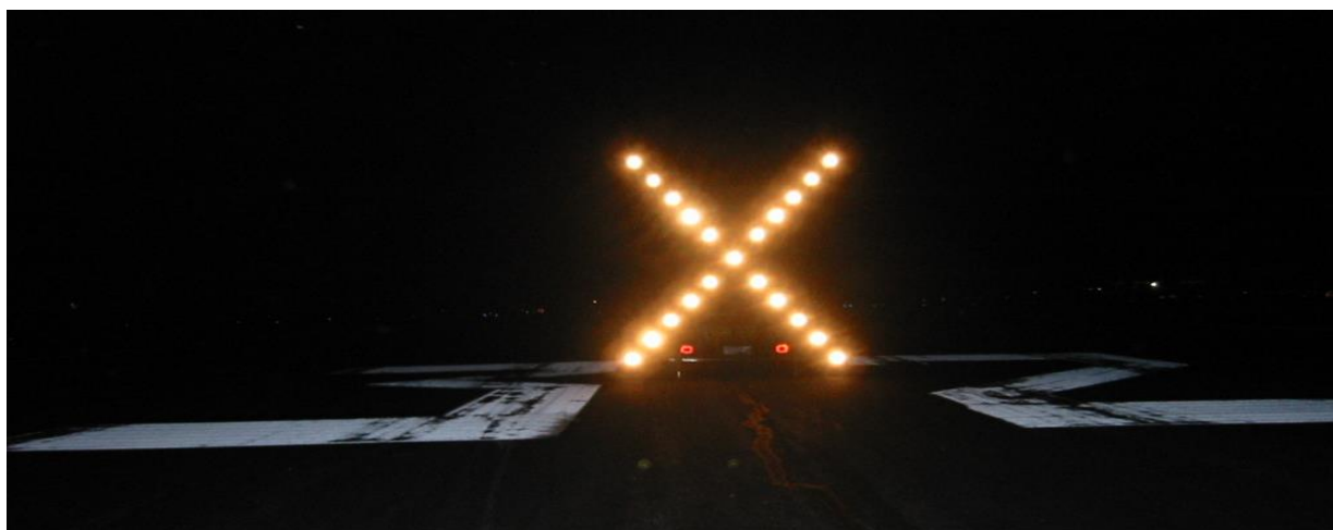
Figure 2-7. Lighted X at Night
